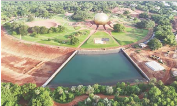
Before the cyclone: The Matrimandir Lake section 1 is almost full, while section 2 (left) has been dug and awaits the lining. The Lego Block wall between them broke.
