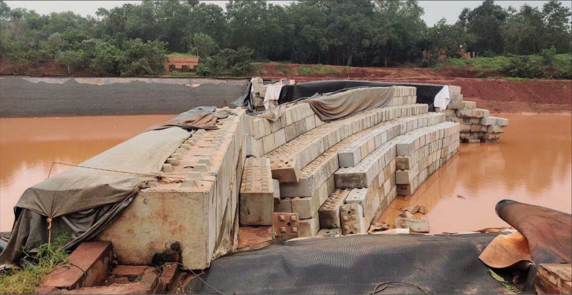
The ‘Lego block’ wall between sections 1 and 2 of the Matrimandir Lake broke in the middle and at the banks
